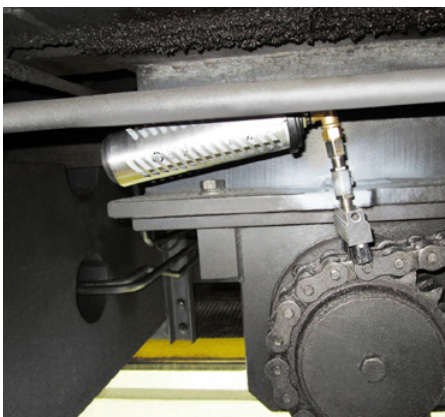
The 250 ml simalube lubricator lubricates the chain drive of a railway crane. The dispenser is also protected by a protective cover.
